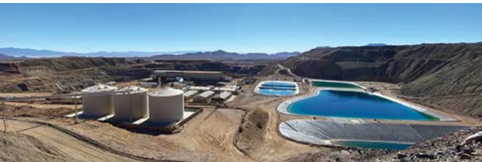
Johnson Camp has a 25 million lb/y SX/EW plant, and pregnant leach solution and raffinate ponds. (Photo: Gunnison)
