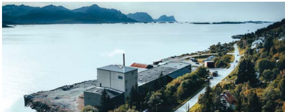
Sitting on Norway’s Senja Island, the Skaland plant produces about 10,500 mt/y of graphite. (Photo: Skaland)
