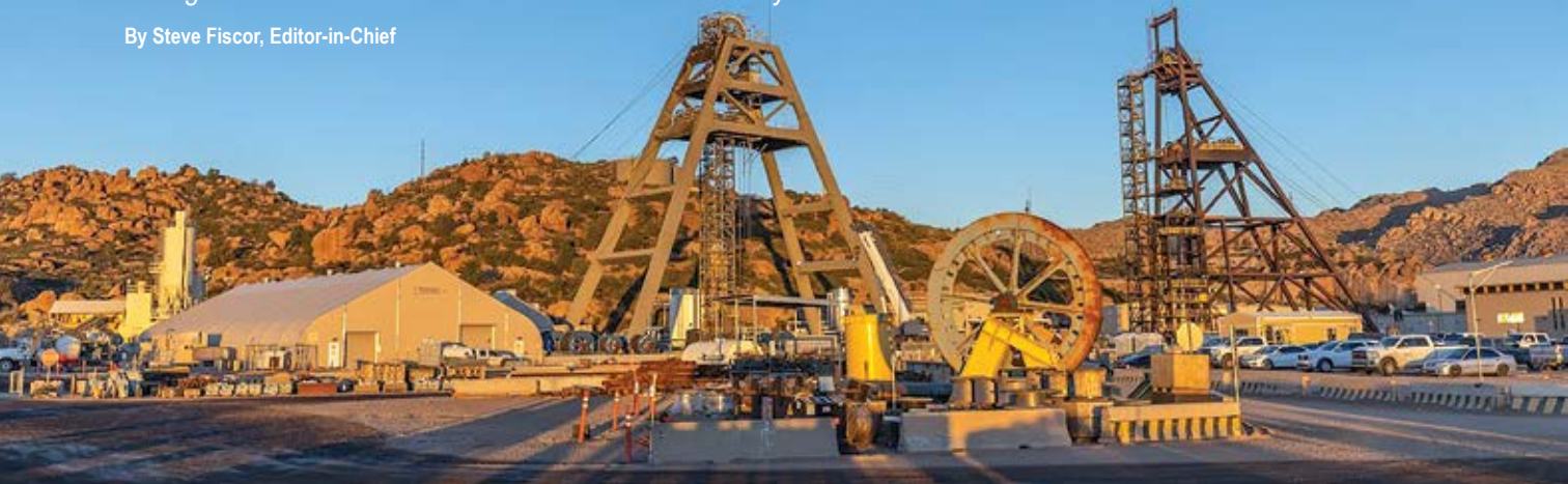
The No. 10 (left) and No. 9 headframes tower over the Resolution project, located near Superior, Arizona. (Photo: Resolution Copper)
